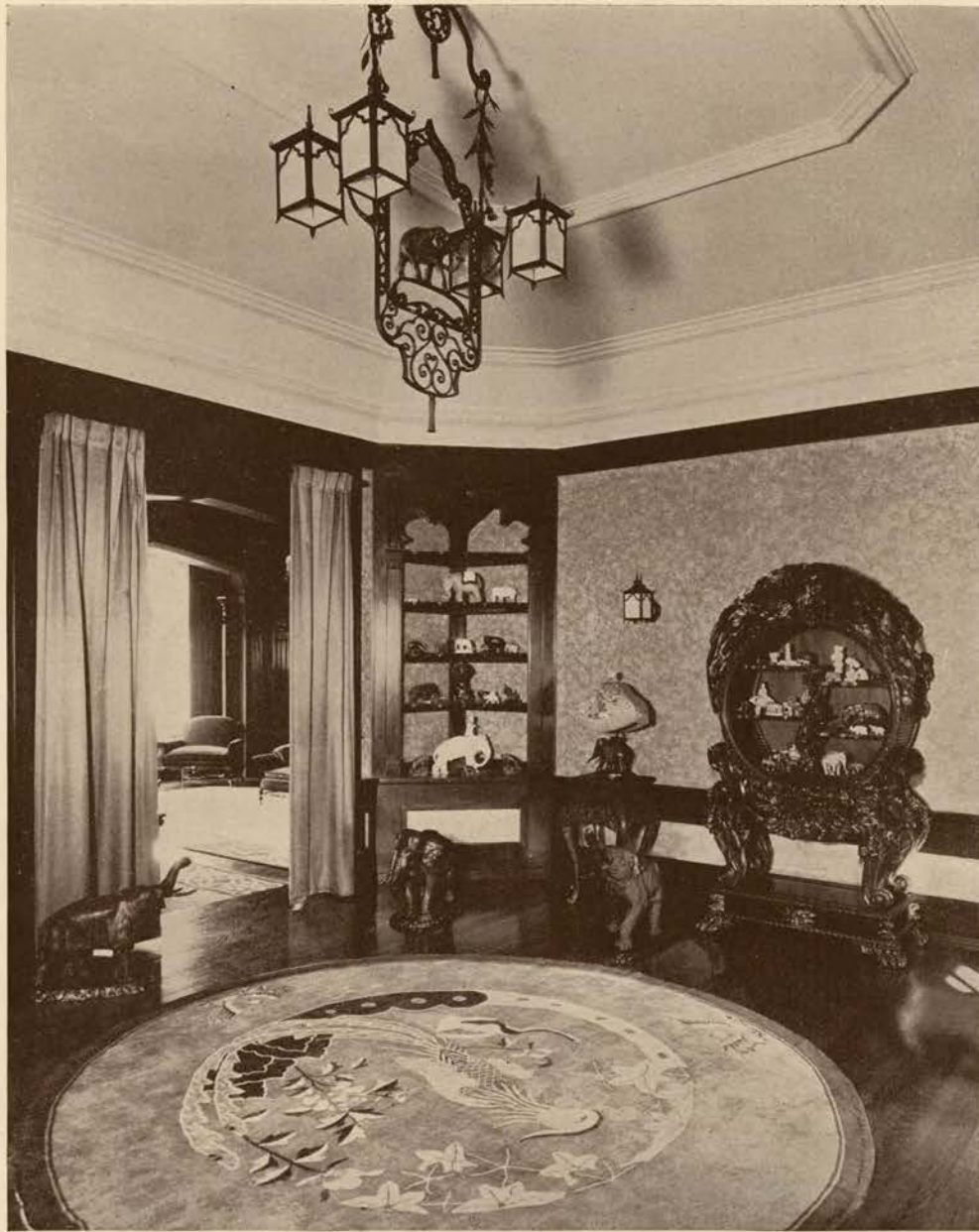
DETAIL of BUILT-IN CABINET in ELEPHANT ROOM
